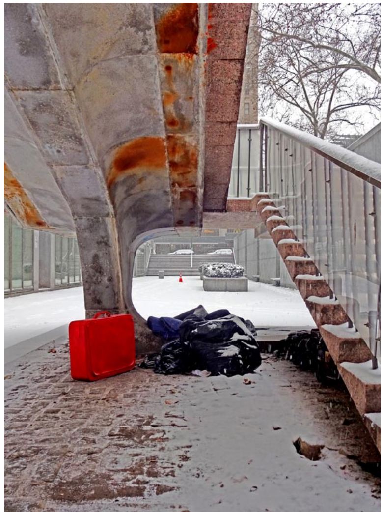
Government subsidised housing: The overflow annex.
