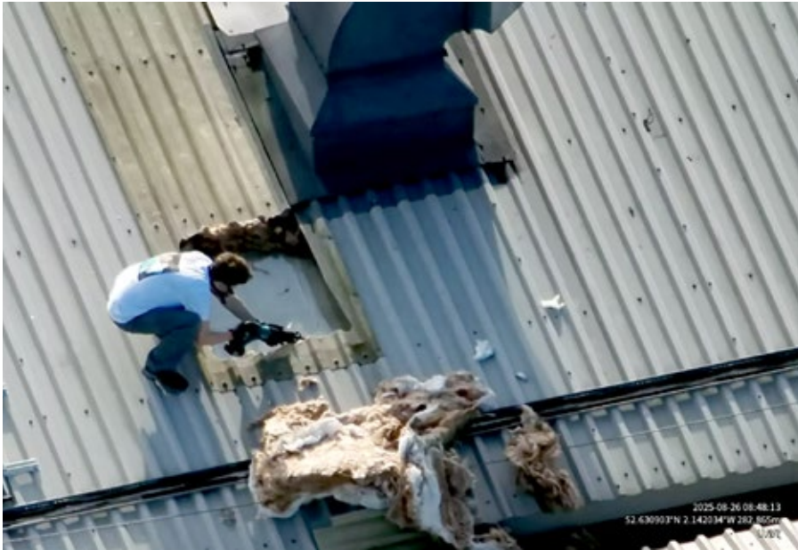
PRO-PALESTINE: Activist cuts through the roof of Wolverhampton arms factory
