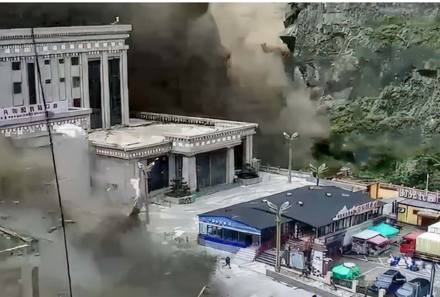
LIKE LIQUID CONCRETE: Surveillance footage shows people fleeing before a mudslide hits Gyirong Port, one of the main border crossings between Nepal and Tibet. At least 384 were killed during the disaster
